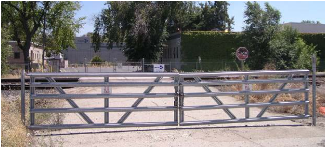
Photo 3.10: Trevarno Road at-grade crossing View: Facing south toward Hexcel Corporation facility Opportunities: Existing at-grade crossing could possibly be used to switch trail from south to north side if a south-side trail is feasible between this point and First Street. Constraints: Operating restrictions on at-grade crossing may not accommodate increased crossing volume if this became a trail crossing. There would be significant crossing improvements and signalization needed to utilize this crossing, and it would be subject to CPUC approval, which is generally not supported.
