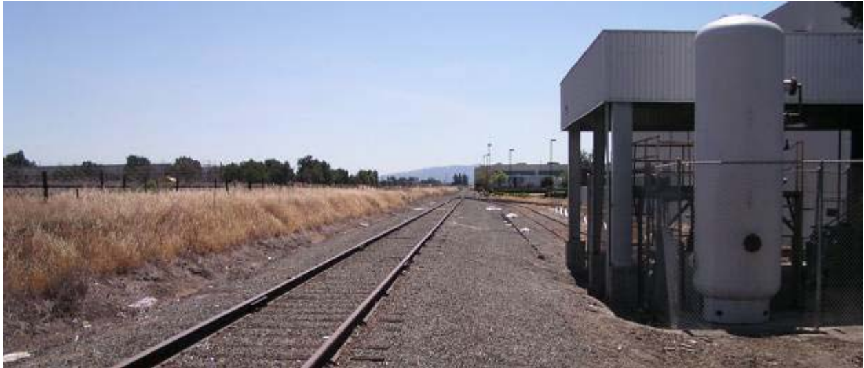
Photo 4.7: North (spur) rail corridor south of Las Positas Road, west of Greenville Road View: Facing west (toward Vasco Road) Opportunities: Wide swaths of open land south of existing track. Constraints: a) Several buildings along north side have features close to the tracks, served by sidings. b) Potential High Speed Rail/expanded freight corridor. Coordinate with HSR cross section. Figure 4-4, Appendix
