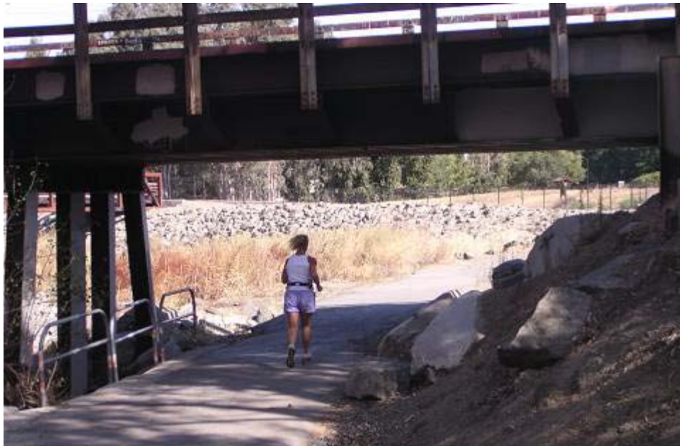
Photo 1.5: Arroyo Mocho Trail undercrossing of active UPRR / ACE rail corridor View: Facing north (Zone 7 service road bridge visible behind rail bridge support at left) Opportunities: Widen trail by rebuilding east embankment (right side of photo). Iron Horse Trail would extend east across Murrieta Boulevard from just south of this point. Constraints: Provide 10' clearance under bridge (12' if equestrian use is anticipated). Flooding during storms may necessitate "storm closure" policy. See Figure: 1-3
