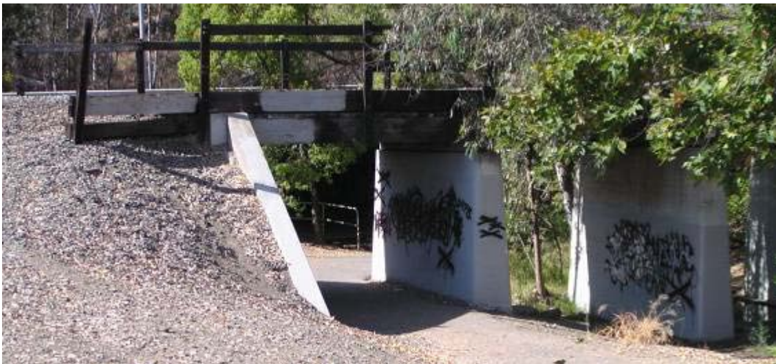
Photo 1.6: Arroyo Mocho Trail under abandoned rail bridge north of Stanley Boulevard. View: Facing south. Opportunities: Remove bridge if not needed for access to area to the west (north of Stanley, south of rail corridor) Constraints: Expense of removing or modifying structure See Figure: 1-3
