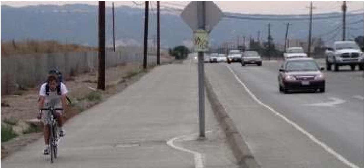
Photo 1.1: Existing Iron Horse Trail along south side of Stanley Boulevard west of Isabel Avenue View: Facing west toward Pleasanton Opportunities: Area to the left (south of Stanley) is planned for water storage lakes by Zone 7. Notes: Zone 7 plans show Iron Horse Trail relocated from along Stanley Boulevard to along the Arroyo Mocho channel north of the rail corridor. See Figure: 1-1, 1-2
