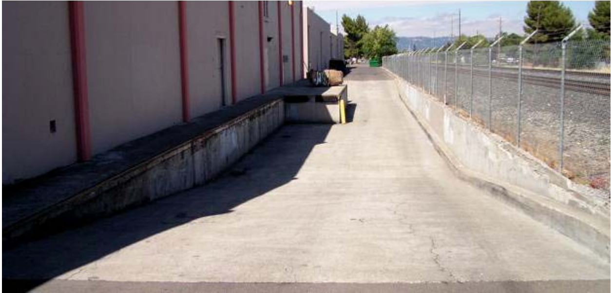
Photo 2.3: Loading dock behind Dollar Tree; railroad corridor to the right. View: Facing west (toward Murrieta) Opportunities: N/A Constraints: No width for Trail. No obvious way to reconfigure loading dock to provide width. If this building is to remain, the loading dock may have to be relocated to a different side.
