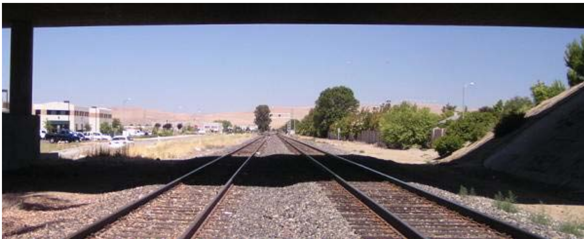
Photo 3.12: Rail corridor east of Mines Road. Contractors Place runs along north (left) side. View: Facing east along centerline of rail corridor, under Mines Road bridge Opportunities: Width is available for a trail along the south edge of Contractors Place. There is an existing EBRPD easement for trail along edge of Contractors Place, north of rail ROW. Constraints: If trail is on south side, the trail would need to be located on UP lands or be routed onto surface streets to connect to lands east of Vasco Road, necessitating easement or ROW acquisition. Bridge supports would need to be modified to provide sufficient width at toe of embankment. See Figure: 3-2
