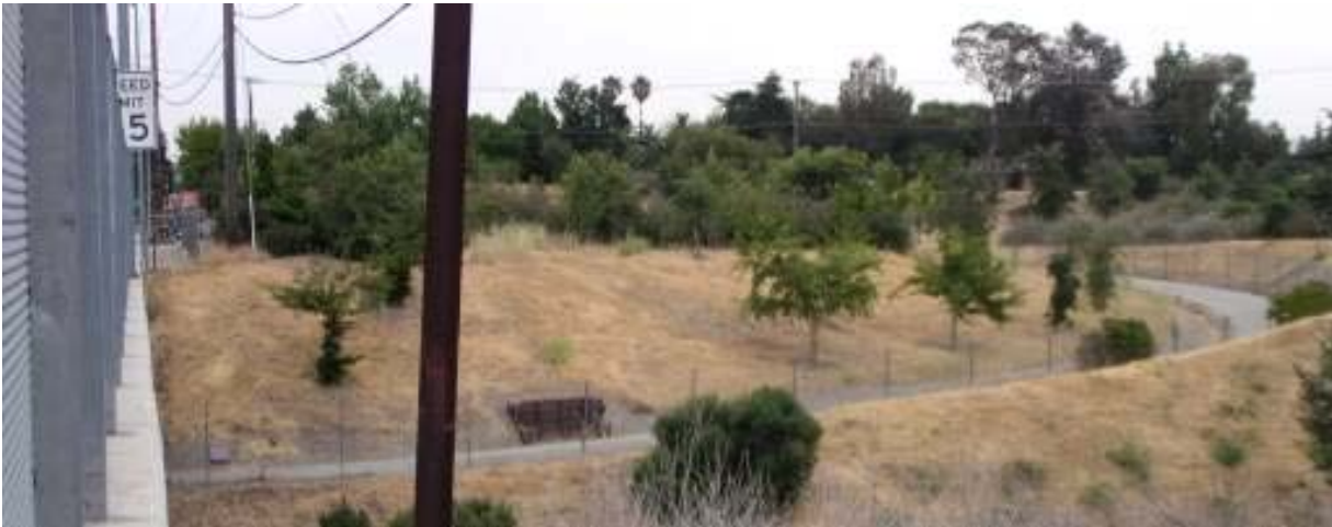
Photo 1.2: Existing loop ramp connecting eastern terminus of existing Iron Horse Trail just east of Isabel Avenue, to Isabel Avenue Trail running under Stanley Boulevard and rail corridor. View: Looking east along south side of Stanley Boulevard bridge over Isabel Avenue. Notes: Isabel Avenue Trail continues along the east side of Isabel south of Stanley. See Figure: 1-2
