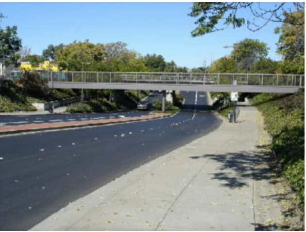
STEEL GIRDER TRAIL BRIDGE AT MURIETTA BLVD.
