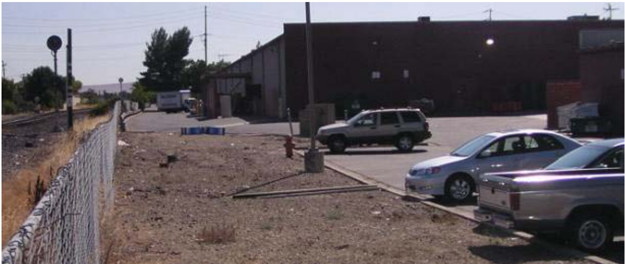
Photo 2.2: Parking lot and loading dock area behind 1070 Stanley Boulevard, just east of the senior apartments shown in Photo 2.1. View: Facing east. Opportunities: Landscape buffer area in foreground has ample width for Trail. Constraints: Configuration of loading dock and driveway behind warehouse currently provides no width for Trail. If this building is to remain, consider: ▪ Moving the loading dock to its west wall (upper right) ▪ Reconfiguring the north (rear) wall loading operations to side-loading ▪ Removing the driveway between the warehouse
