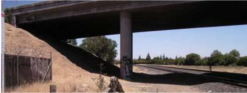
Photo 3.5: North side of rail corridor at First Street overcrossing View: Facing east. U-Haul fence at left side. Opportunities: N/A Constraints: Embankment may need modifications to accommodate trail while providing 25' of separation to centerline of outer tracks. See Figure: 3-1
