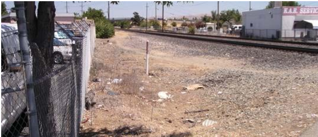
Photo 3.2: East of Junction Avenue (First Street overcrossing visible in distance)
