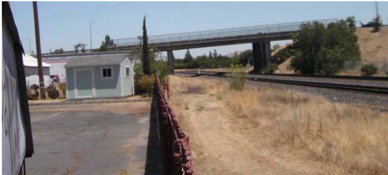
Photo 3.4: First Street overcrossing View: Facing east along north side of rail corridor Opportunities: Ample width for trail to stay 25' from centerline of active tracks, except along closest building to northwest corner of overcrossing (U-Haul) Constraints: Closest building in U-Haul yard may constrain width on north side. See Figure: 3-1
