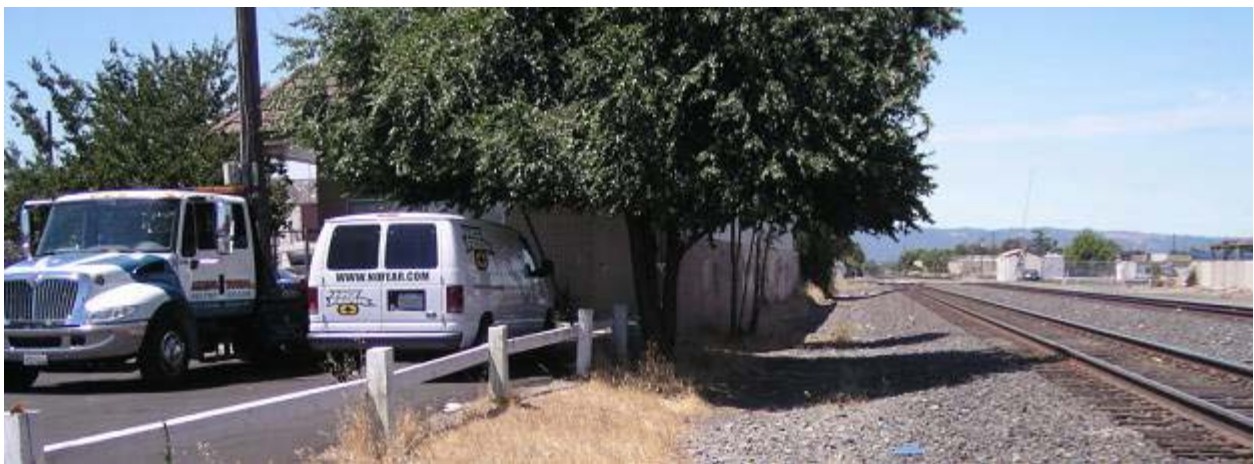
Photo 2.14: Rail corridor between L Street and South Oak Street View: Facing west (toward L Street) Opportunities: N/A Constraints: Existing commercial building (behind wall) blocks trail alignment along rail ROW. See Figure: 2-2
