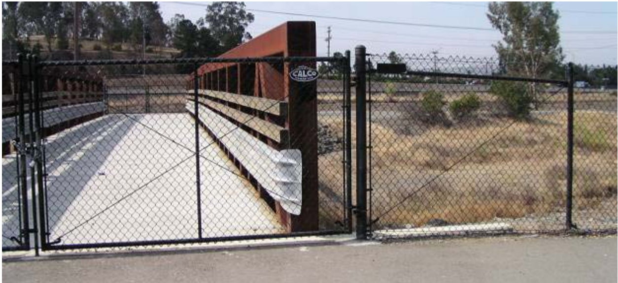
Photo 1.4: Zone 7 bridge over Arroyo Mocho channel just east of Murrieta Boulevard, connecting north and south service roads. View: Facing south from north service road. Rail corridor visible beyond. Opportunities: Trail crossing point across channel if Iron Horse Trail is aligned on south service road. See Figure: 1-3
