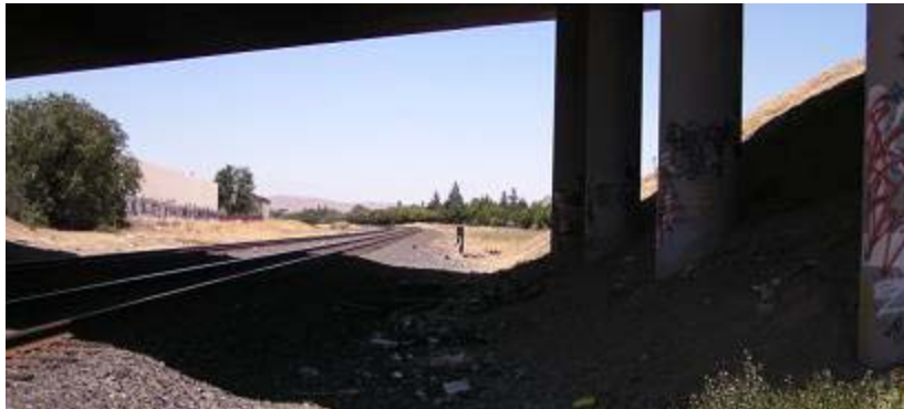
Photo 3.6: South side of rail corridor at First Street overcrossing View: Facing east Opportunities: N/A Constraints: Embankment may need modifications to accommodate trail while providing 25' of separation to centerline of outer tracks. See Figure: 3-1
