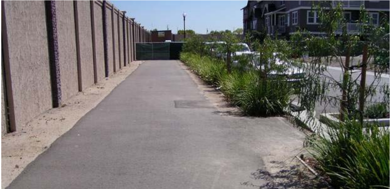
Photo 2.9: Existing trail segment through Railroad Depot condominium complex View: At midpoint of development beside internal crosswalk, facing east (toward L Street) Opportunities: Extend trail along railroad edge when an easement can be acquired from the owner of the NE corner property at L Street, currently occupied by an equipment rental business. Constraints: Business at NE corner of development site currently blocks trail from direct alignment along railroad ROW. Temporary alignment follows project's internal driveways. See Figure: 2-2
