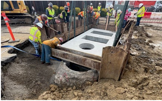
Work on manhole covers on Southfront Rd at First St
