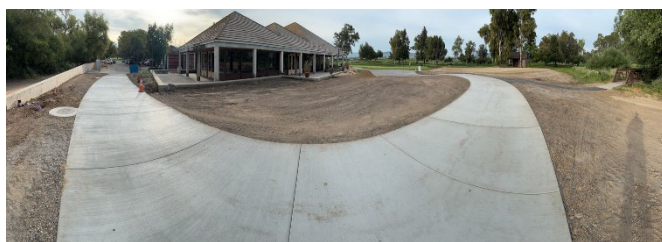
Work completed adjacent to Beeb’s
