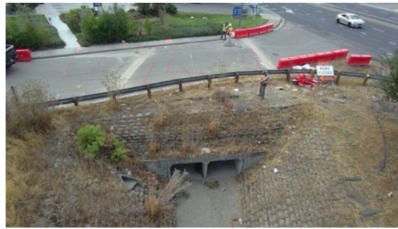
Southfront Rd & First St before installation work
